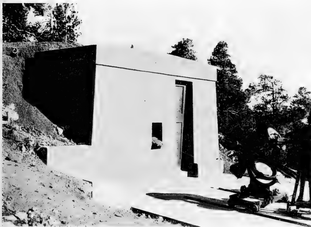
FIG. 32.—Concrete observing tunnel at Table Mountain, California.
